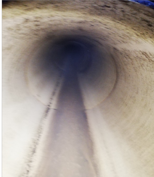
Photo 5: After the application of Microbe-Lift. The wastewater pipeline in Jægergårdsgade is solid build-up-free. (Credits: Aarhus Water, December 2019)
