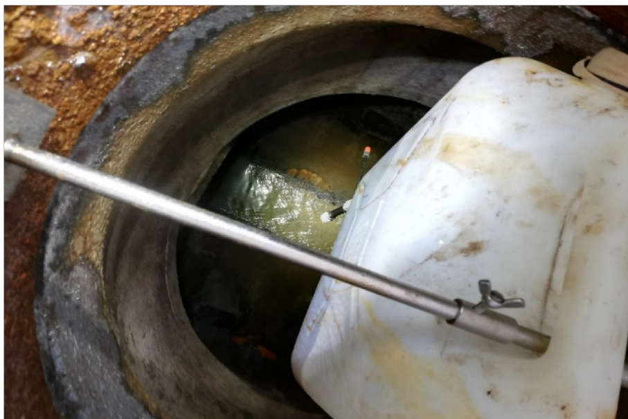
Photo 4: The dripping method used to introduce the solution well in the wastewater pipeline in Jægergårdsgade (Credits: Aarhus Water, December 2019)
